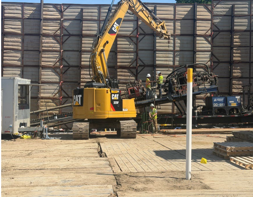
Facing north near MP 2.4, continuing the pilot hole on HDD P4-5
