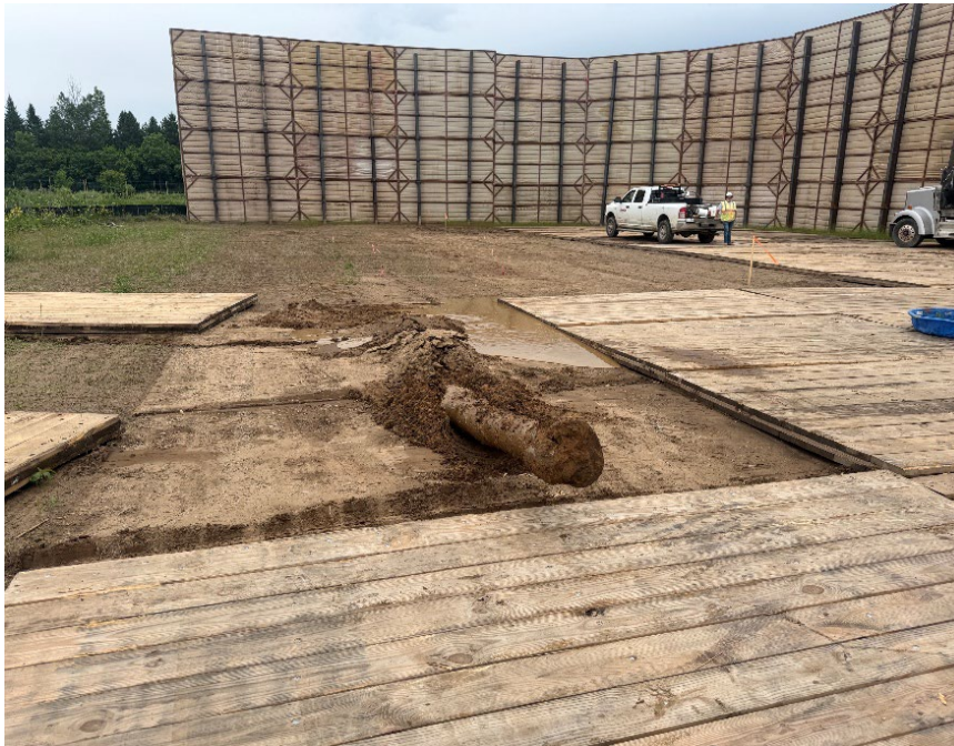
Facing east near MP 2.4, completing the pilot hole on HDD P4-5
