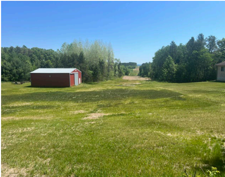
Facing east near MP 2.55, landowner has removed straw wattles and mowed, in the background a mosaic of tilled agriculture and restored pasture are visible on the right of way
