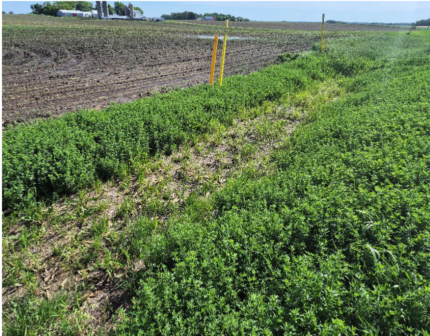
Facing northeast at MP 31.95, erosion control blanket (ECB) functional revegetation at 55 percent of adjacent vegetation
