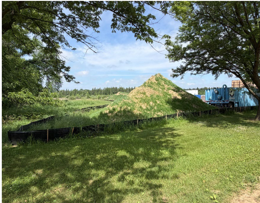
Facing west near MP 2.4, topsoil stockpile stabilized with hydroseed
