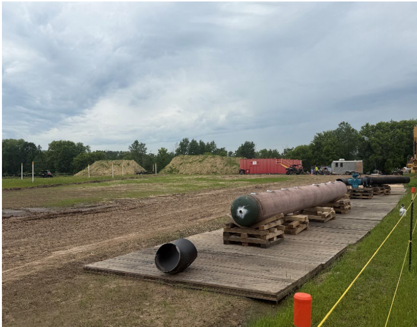
Facing southwest near MP 3.42, welding continues
